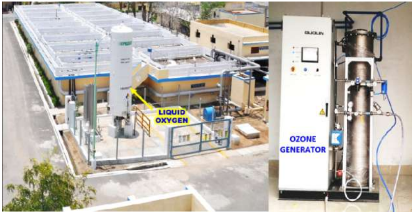
Fig.3: Addition of liquid oxygen & Ozone at high cost for control of Sulphide & survival of aerobic biomass
